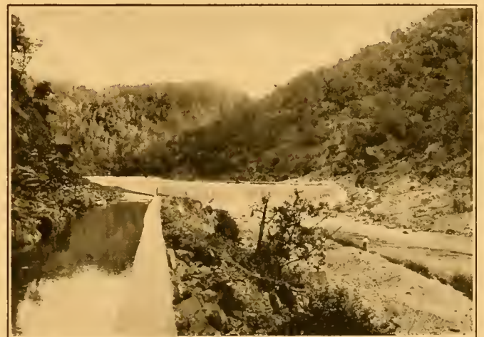
SOURCE OF WATER SUPPLY FOR FAIR OAKS AND VICINITY. DAM OF THE CALIFORNIA CORPORATION
